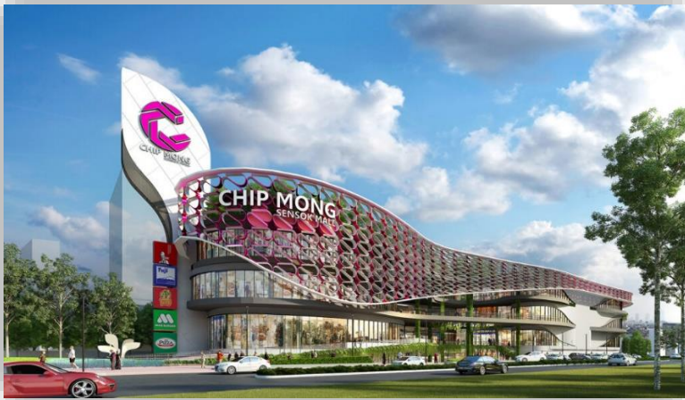
○ CHIP MONG SENSOK MALL PROJECT
